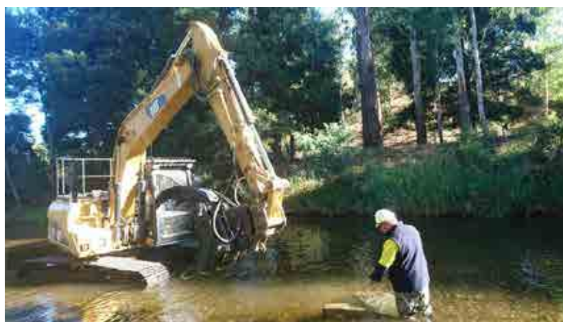
Figure 6. Boulder seeding in the lower Howqua River undertaken by the Goulburn-Broken Catchment Management Authority.
